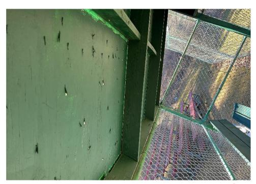
The picture of inside of dugout shows exposed nails. Still not sure how we're going to address this problem. Last picture is of some type of broken box with wires that come out. Not sure what it goes to but could definitely use some attention.
